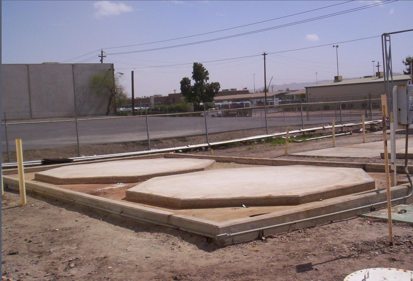
Foundation for new tanks
